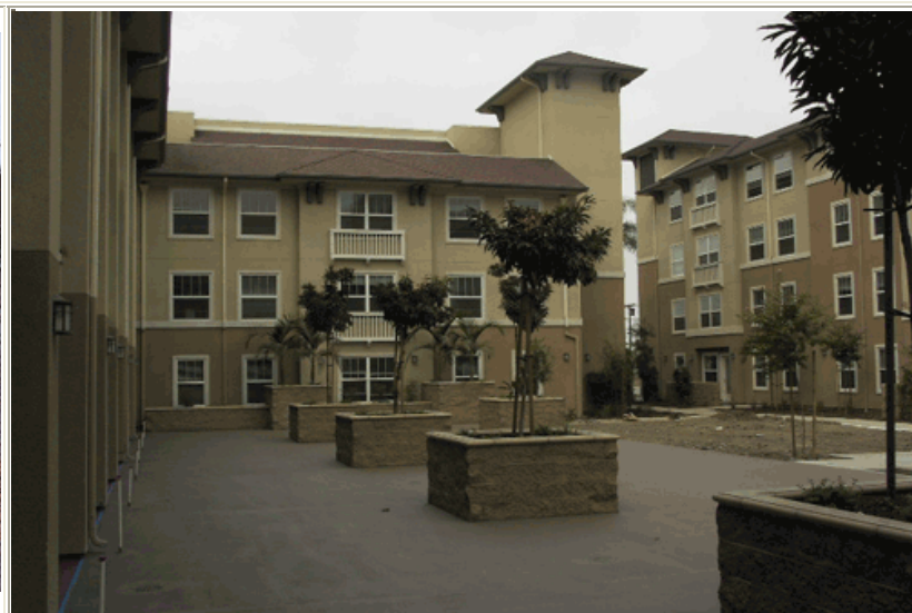
Las Brisas after redevelopment.
